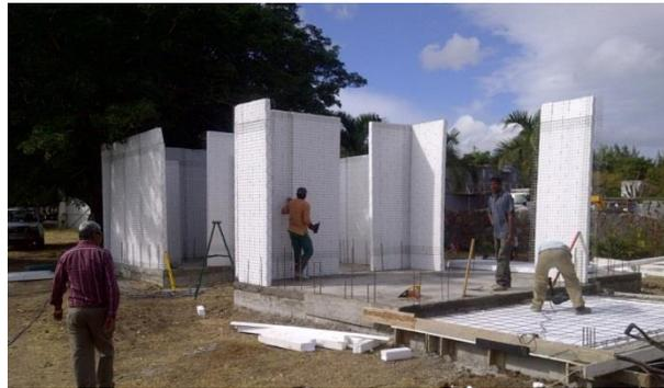
An AP panel is an engineered steel wire mesh assembly system of the most advanced technology in reinforced concrete. This combination of a three dimensional structural wire panel, stucco and polystyrene core have made possible these prefabricated panels of exceptional durability and strength, at a fraction of the weight of cement blocks or brick masonry.
