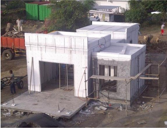
Uptake in Mauritius has been particularly good, despite its location in a hurricane zone, Mauritians realise the strength of the system and have embraced its benefits wholeheartedly. The interlocking EPS panels, set in mesh, can be clearly seen in this image. Plastering has begun on outside of the room on the right.
